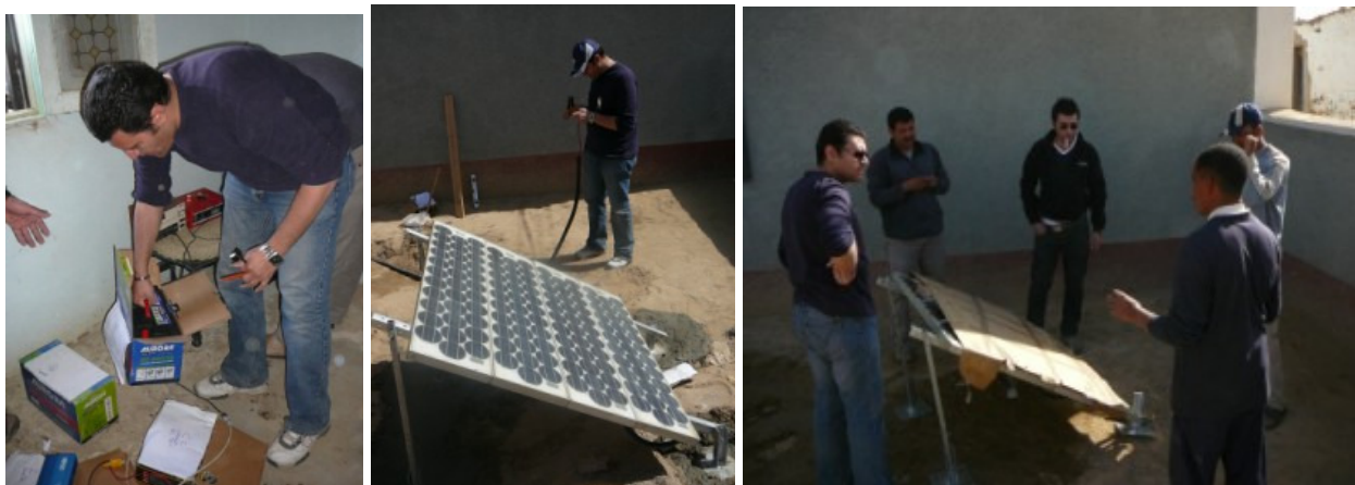
Figures 1-3: Installation of the solar system in Abu Minqar. RISE decided to recycle 30 year old panels for this project that were still working at 70 percent capacity.
